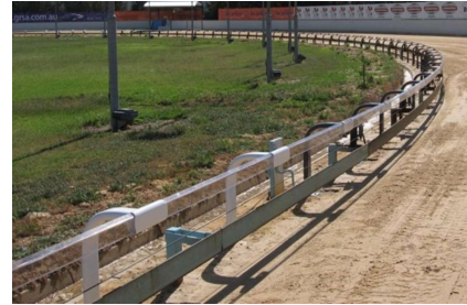
Traditional steel post & lure rail system with plastic safety rail used in SA
