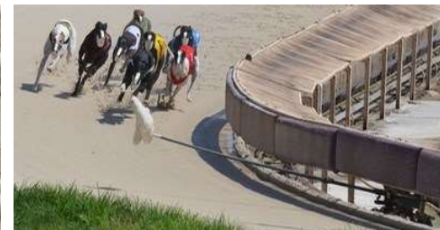
USA steel inside barrier system, covered with foam padding and cableless lure operating on rails below the inside barrier
